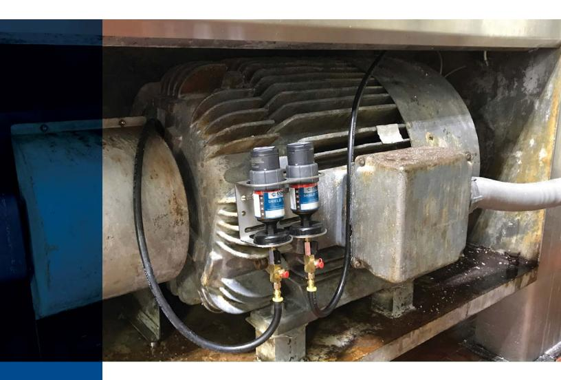
Extend Bearing Life with Automatic Lubrication **SHIELD LUBRICATORS**
